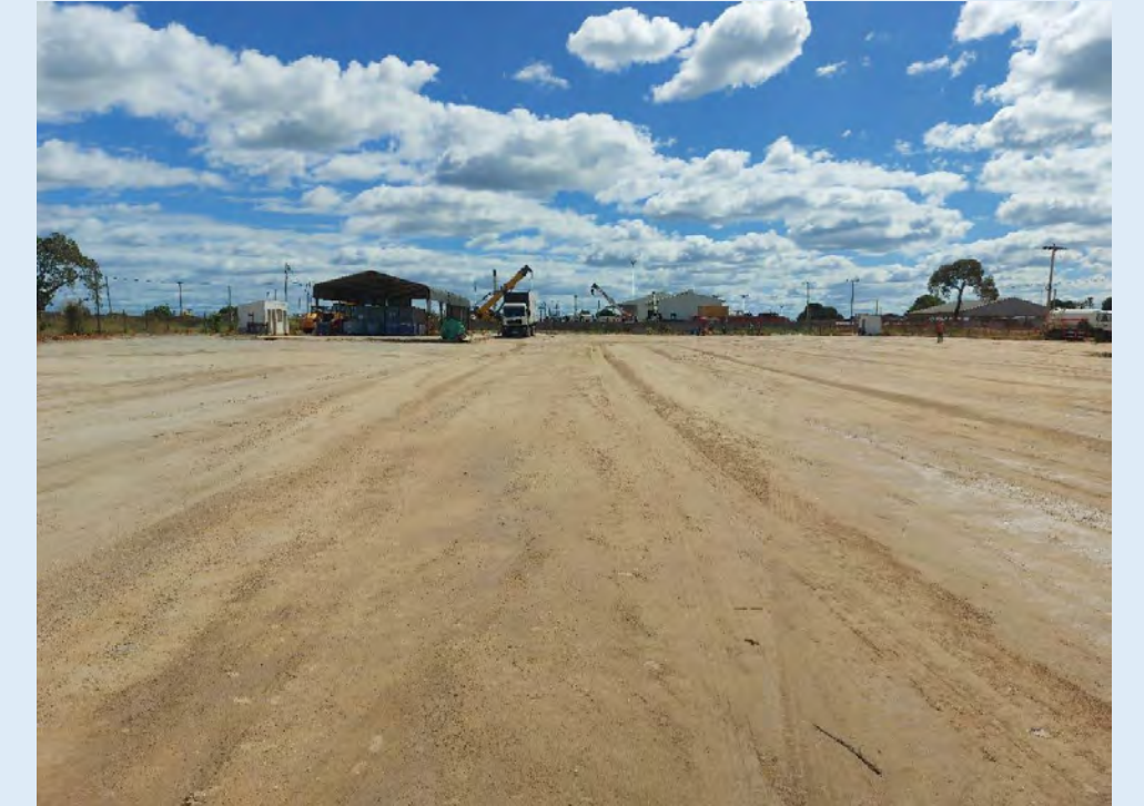
Prepared area with crusher run 12,474 m2 (100mm thick)
